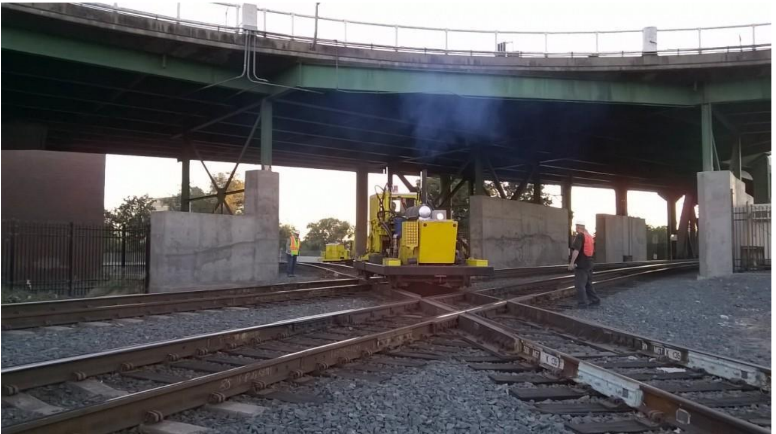
Dave pilots the tie-shear over the UP Main
