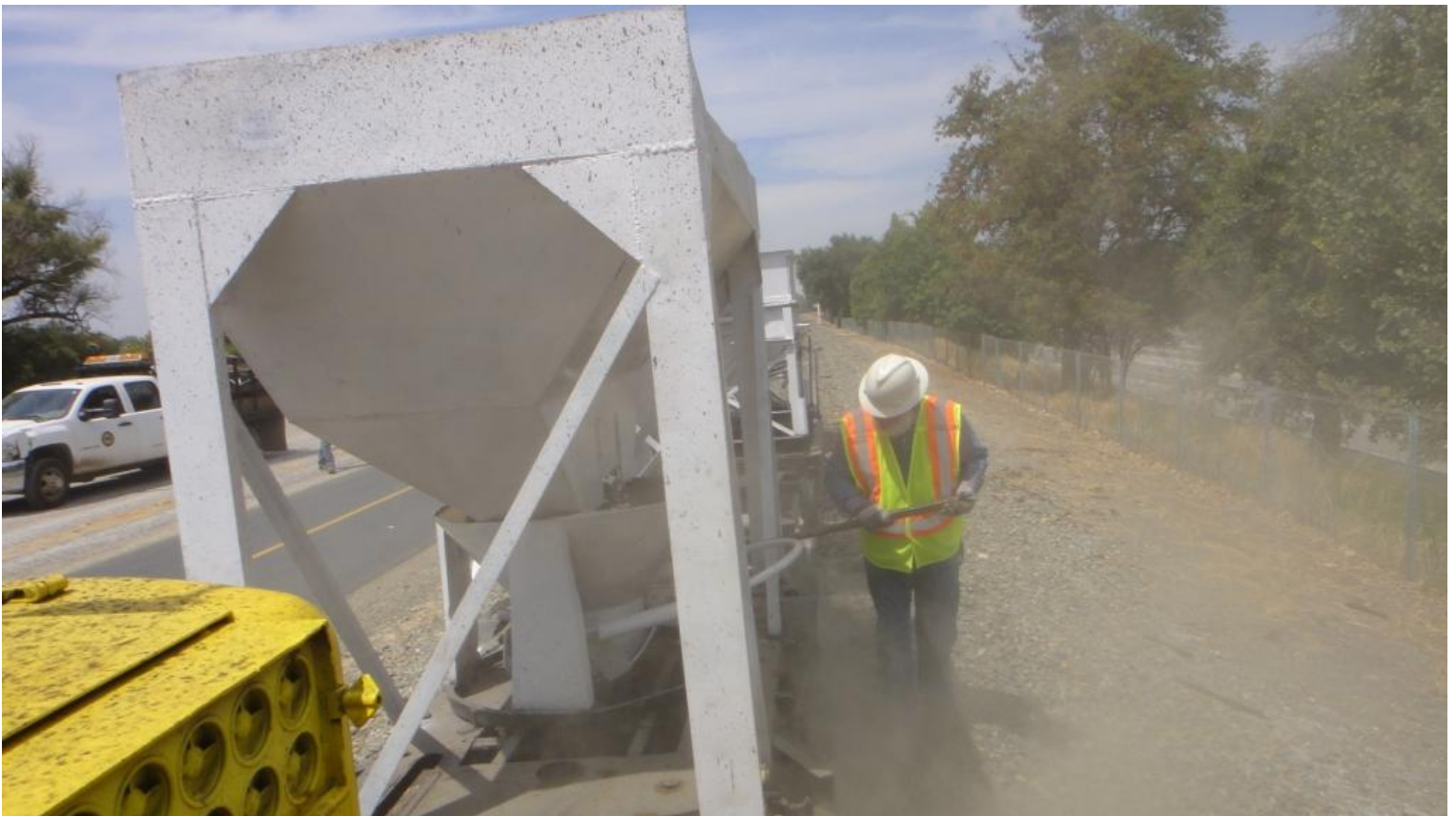
Frank working in a fog drops rock between the rails with the center-dump hopper (which, by the way, was built by Cliff Hayes)
