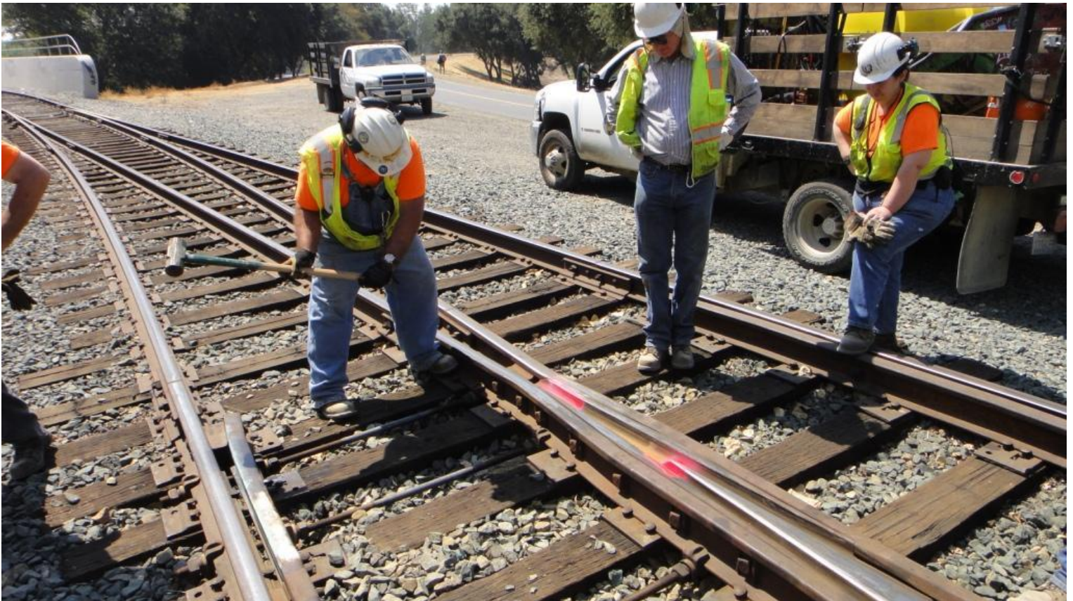
Mike F. uses the sledge hammer to shake-up the frog bit
