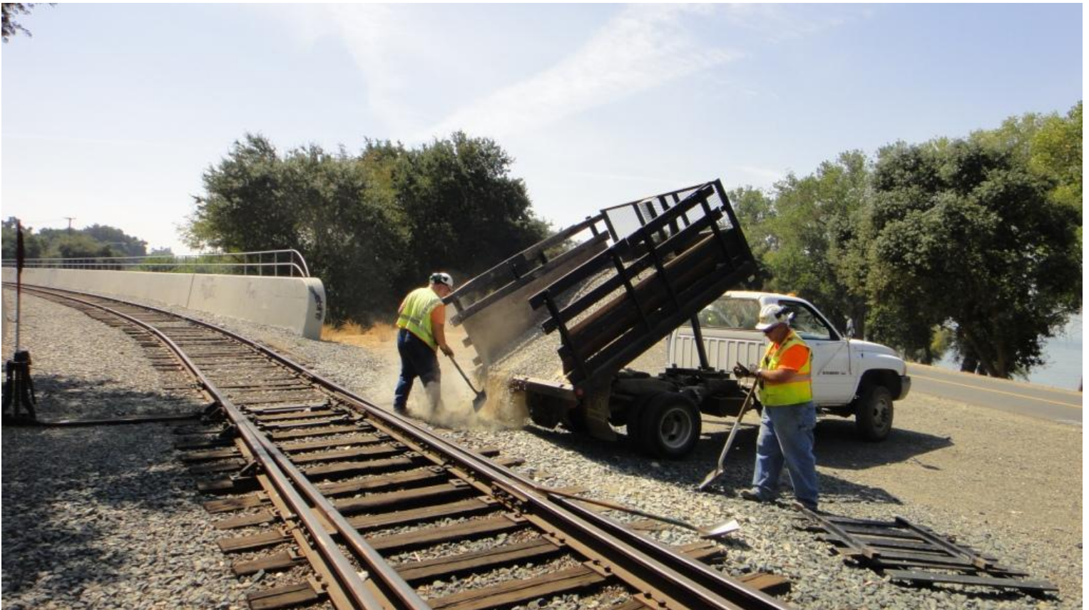
Near Switch 20, Frank W. and Mike F. level the area where brakemen step off the locomotive when it is facing south
