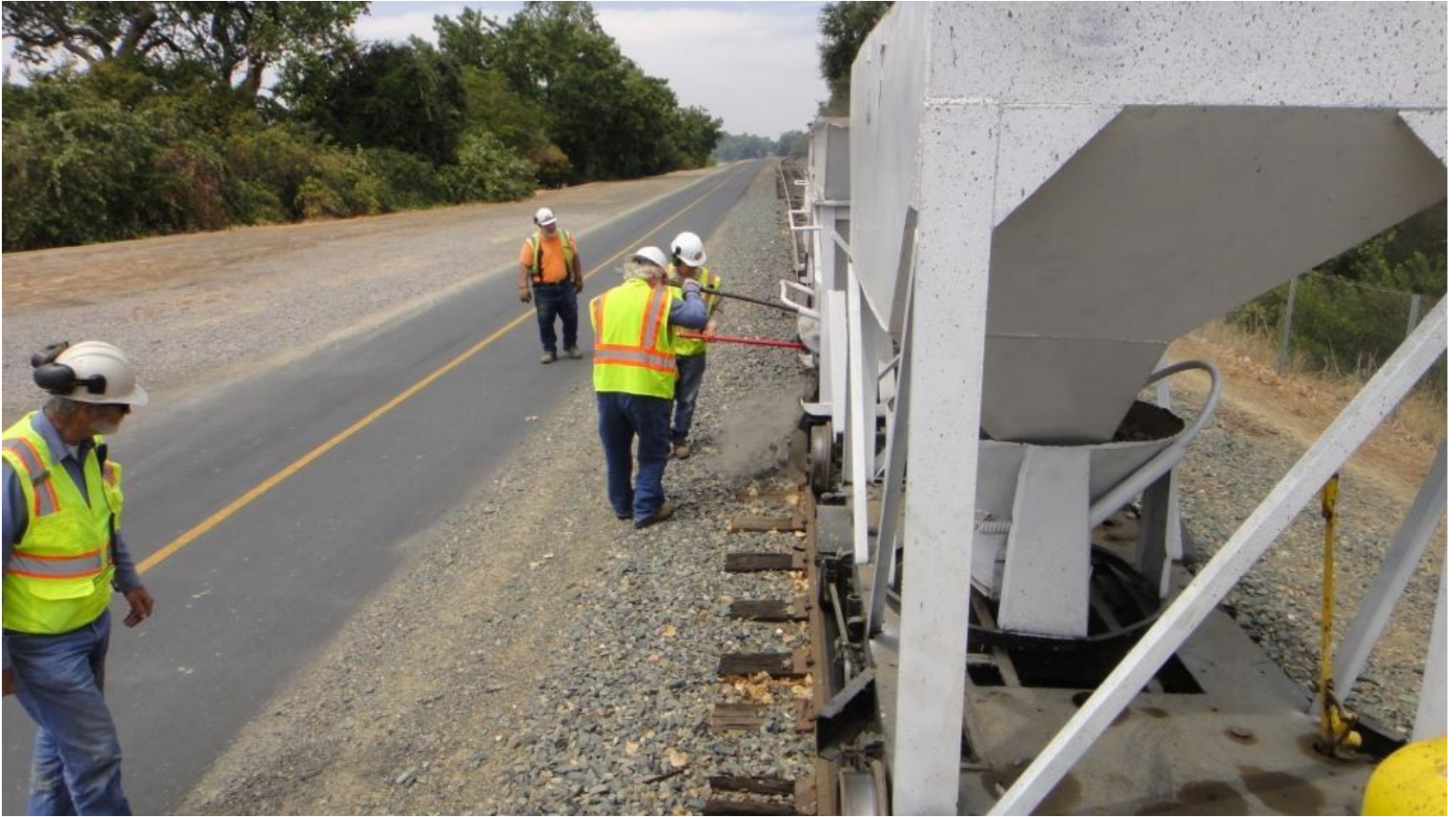
...Which Mike W. and Frank S. lay out along the west rail near Mile Post 2.65
