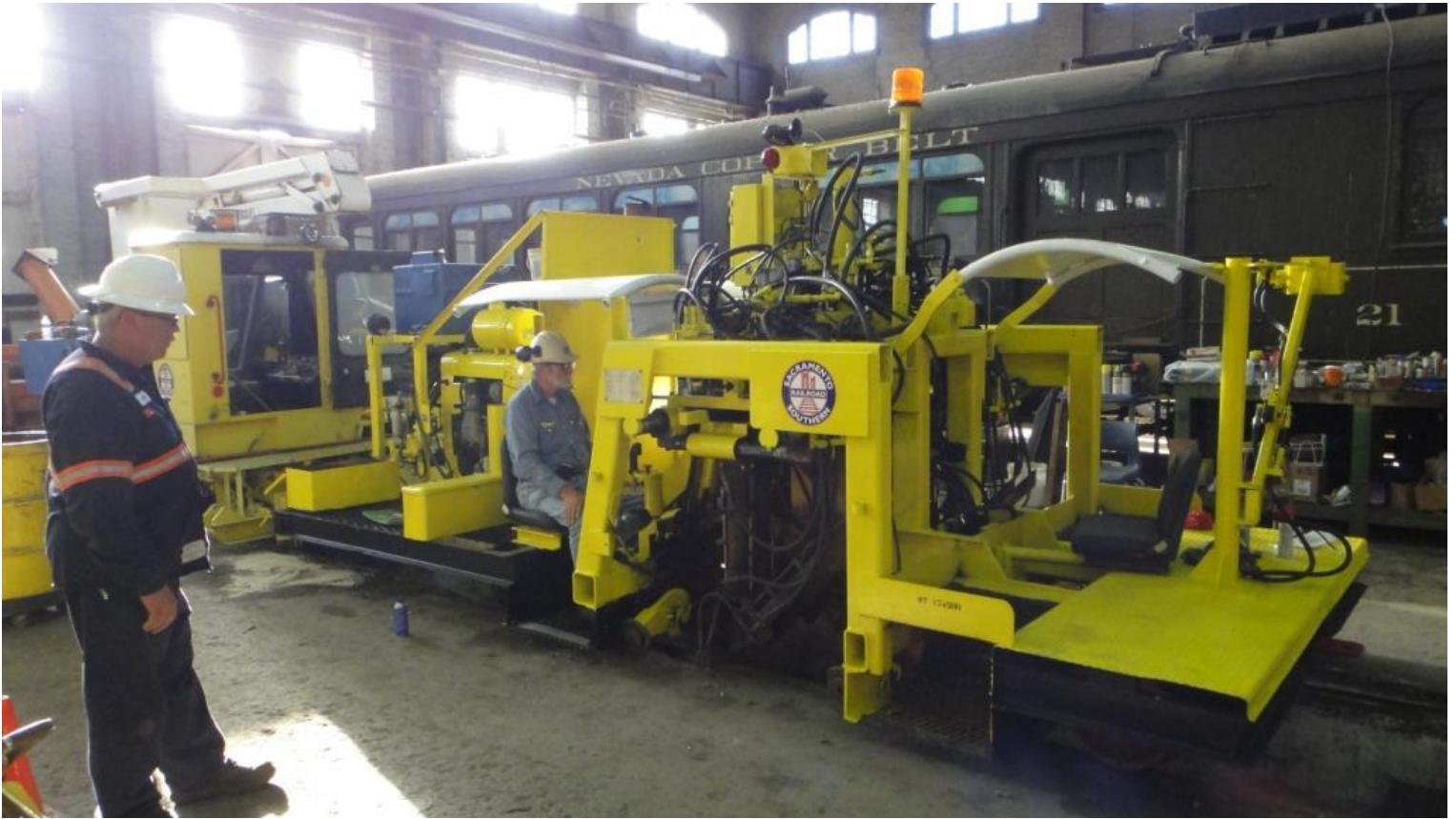
After Mike H. installed the new solenoid on the Super B, the brakes release on command and no longer require manual override
