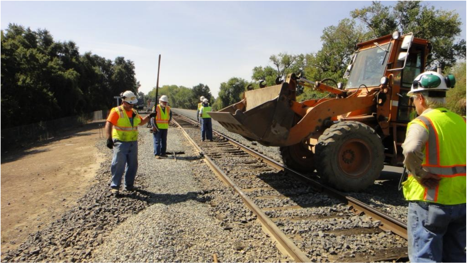
Frank W. in the loader brings in more rock to lay on the brakemen's landing strip at Switch 17
